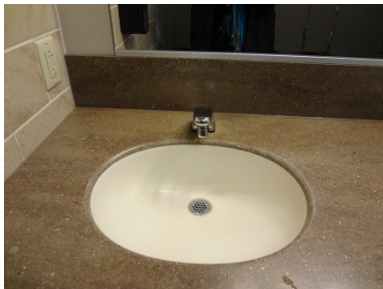
Figure. 22. Demonstration of motion-sensored faucets in public bathrooms
