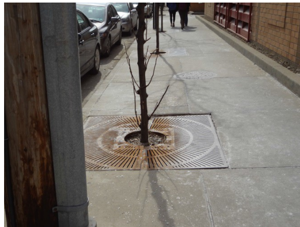
Figure 26. Treebox on Atwood in front of generator facility
