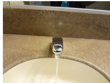
Figure. 22. Demonstration of motion-sensored faucets in public bathrooms
